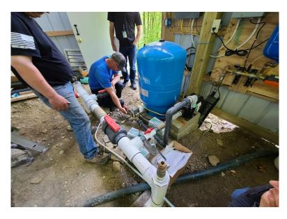
Photo showing a unique constant pressure manifold system at the reservoir site of a seasonal campground.
